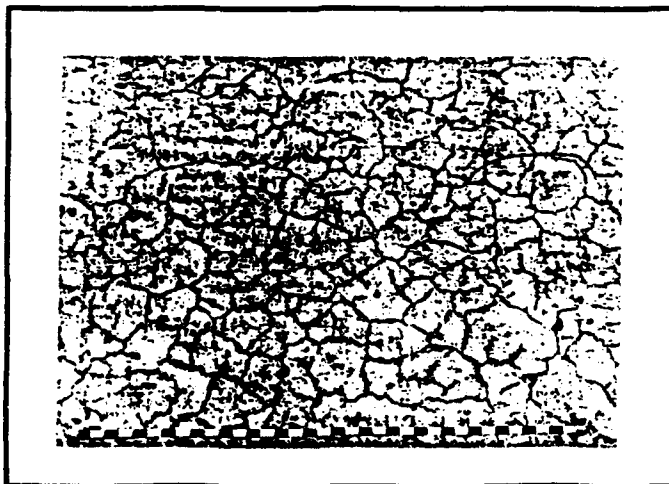
Figure 2.2 Map Cracking (Reference 4)
